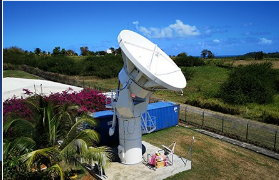
Calian SED (Saskatoon, SK) Composite Carbon Fiber Antenna (6- and 10-m) for Q/V band satellite communications (March 2019)
