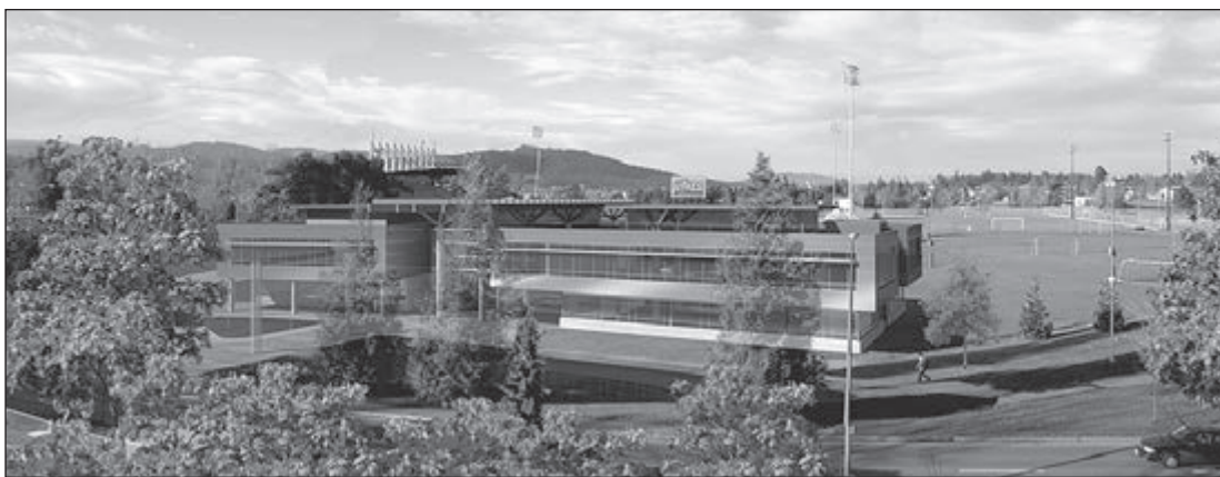
Architectural illustration of the Support Services Building (view from Ring Road). Sustainability features will include a stormwater management system incorporating landscaped retention ponds near the building entrance.
