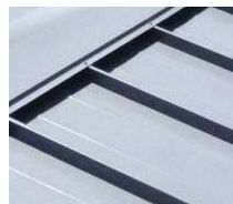
STANDING SEAM ROOF
